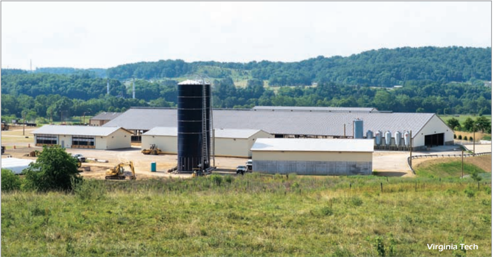
VT Dairy Science Complex - Kentland Farm
