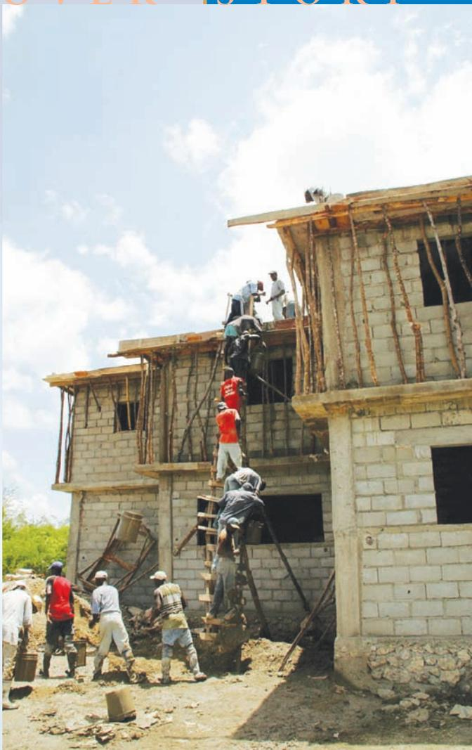
The concrete bucket brigade goes up a ladder as a new building is constructed in Jamaica
